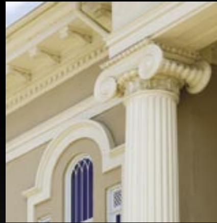
PULASKI COUNTY COURTHOUSE—HAWKINSVILLE, GEORGIA. IONIC COLUMNS WITH GREEK ERECTHEUM (WITH NECKING) CAPITAL.
