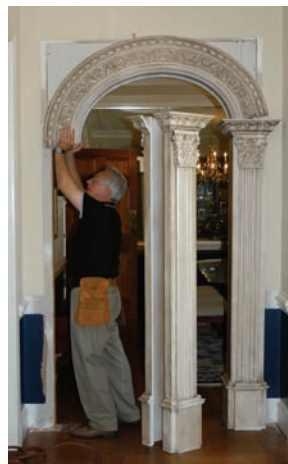
Place Arch Head and Columns
