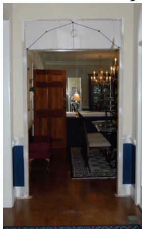
Drop, Mark and Cut Sheetrock
